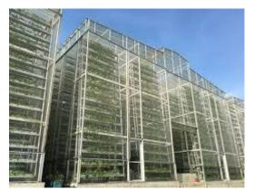
Sky Greens, established in 2012, is known for its innovative vertical farming system, which utilizes hydraulic-powered, rotating tiers to maximize sunlight exposure while minimizing energy consumption. Located in Singapore, the farm provides fresh, locally grown vegetables to the urban population.
